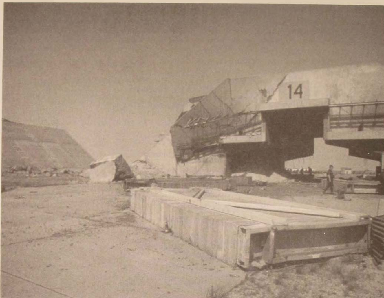
The Iraqi air force had essentially "hunkered down" to protect itself. The coalition undertook a major effort to find and destroy the sheltered aircraft so that the Iraqis could not use them later in a surprise "Tet-like" offensive. Here, steel blast doors from an aircraft shelter have been blown across the tarmac after a coalition air attack.
